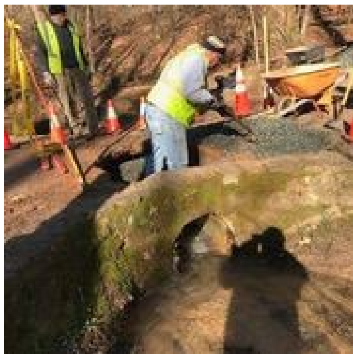
Roadbed collapses over culvert on Fire Rd.. Emergency repairs completed to insure safety of hikers and horseback riders.
