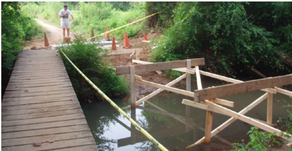
The narrow bridge over John Ward Creek on the west side of the Park was a safety hazard. Horses waded through the water to the right of the picture but not at high water when the creek rose up to the level of the bridge. This photo was taken after the concrete abutments for the new bridge were poured and after Ray Scott built the cambered falsework to hold up the bridge during construction.
