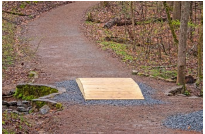
Finished emergency project on Noses Creek Trail. Photo by Fred Feltmann
