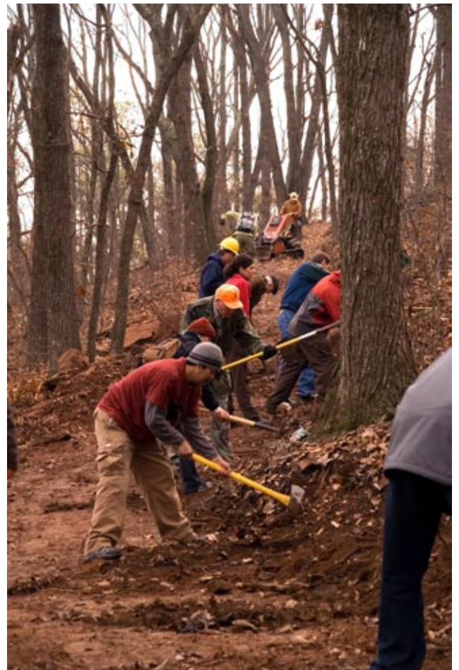
WORKDAY ON THE NEW TRAIL SECTION - 1/12/08
